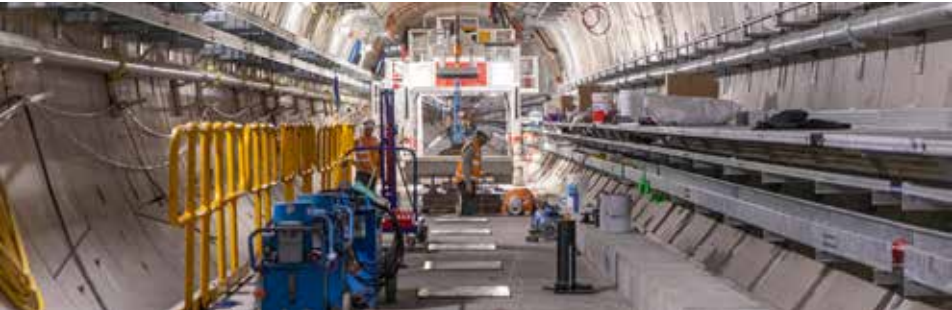
▼ Crews installing the floating slab track through the Metro Tunnel.
