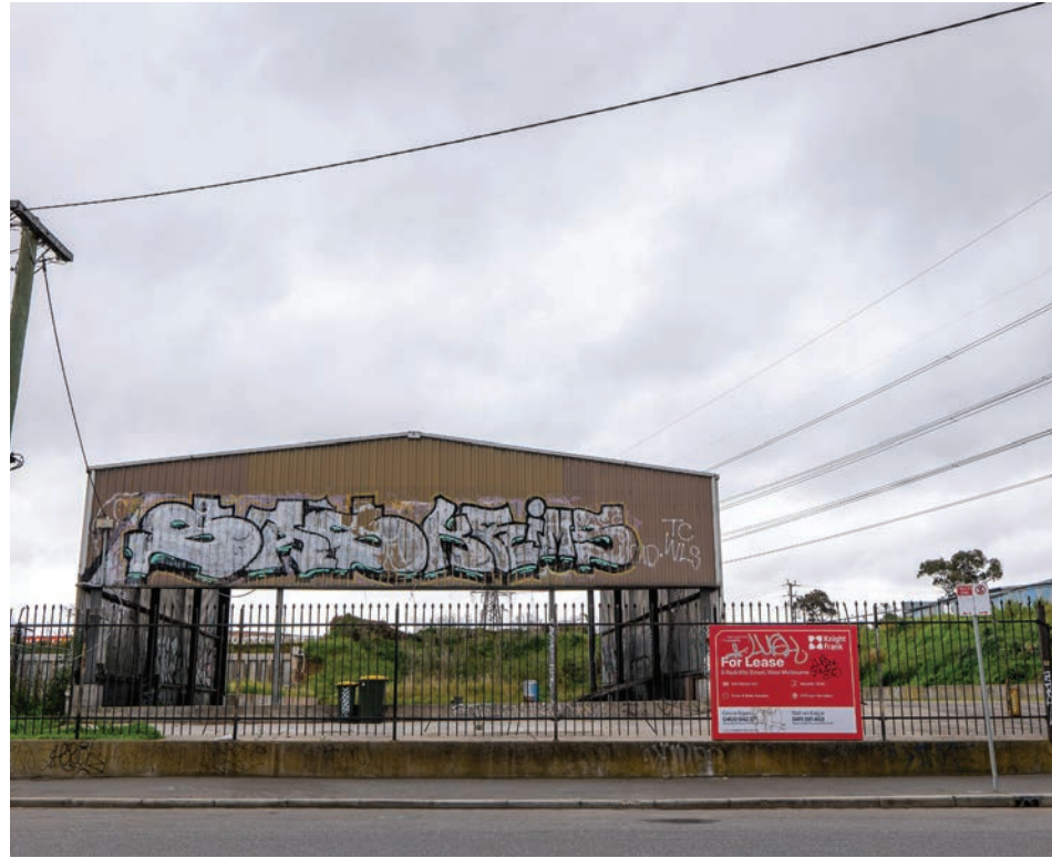
▲ The site at 8 Radcliffe St, West Melbourne.
