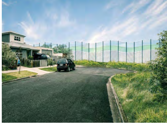
▲ An example of a potential noise barrier being promised to a Le Fevre St in Spotswood as part of the project, which according to the WGTP, currently experiences “up to 70 decibels” - above the 63 decibel noise limit.
