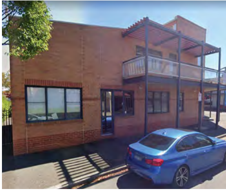
▲ 30-38 Gatehouse Drive, Kensington
