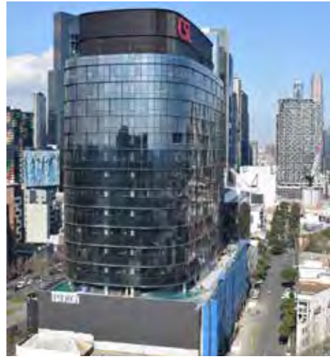
▲ The nearly complete new CSL headquarters near Haymarket roundabout.
